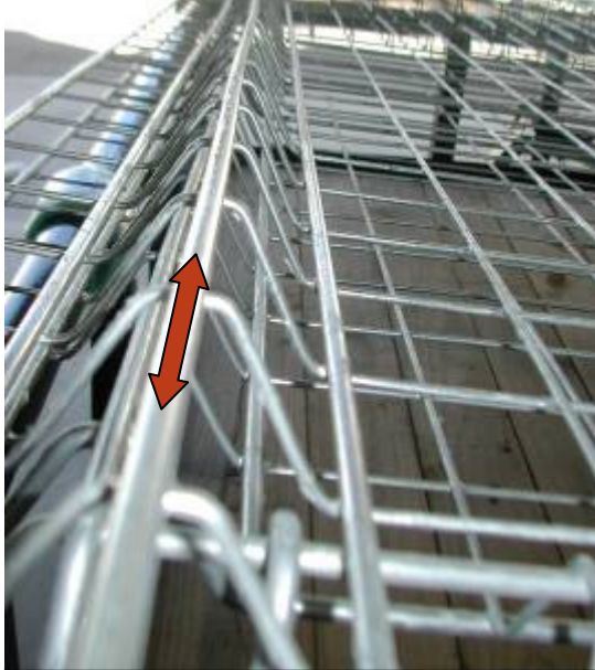
1. Each V has a straight wire the length of the panel creating a set of "rail tracks".
