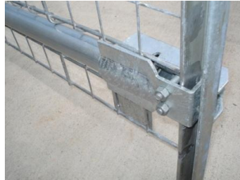
Gate ell installed weld to tube.
